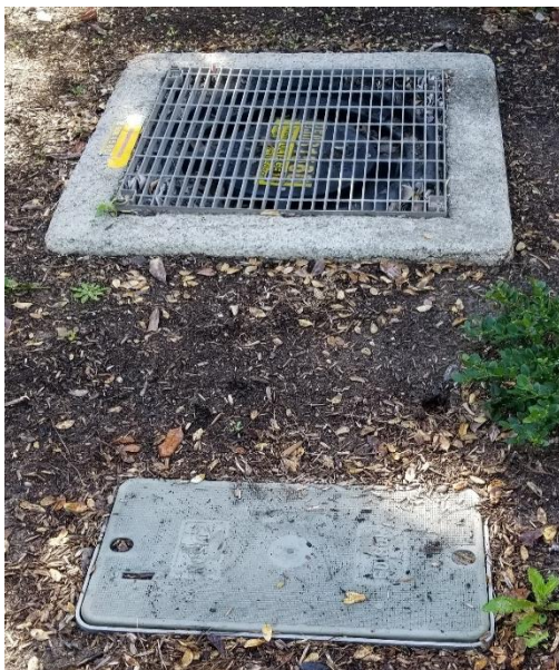
Figure 6: SCE Subsurface Transformer Installation
