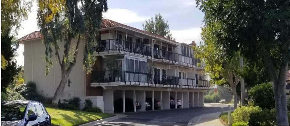
Figure 15: Under-Building Carports at C327
