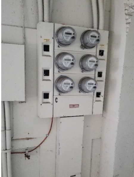
Figure 9: One of the Six-Meter Residential Panels at C219
