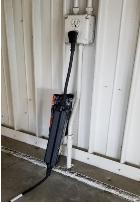
Figure 14: Level 1 EV Charger in United Laguna Hills Mutual Residential Area
