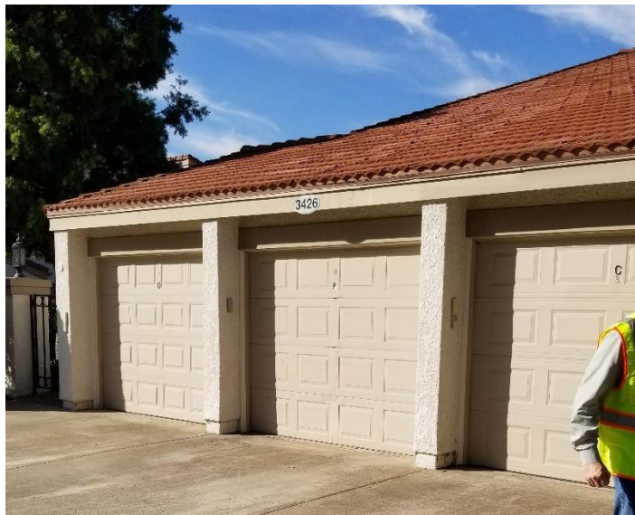
Figure 14: Detached Garages at C344
